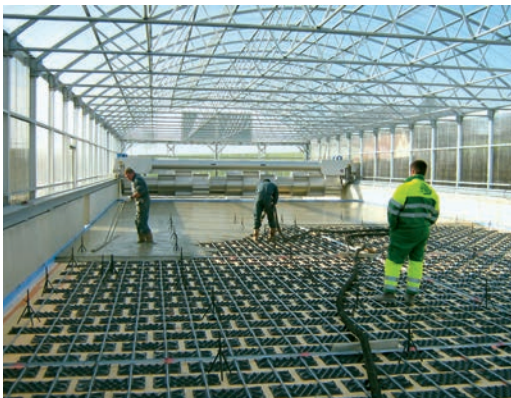
Higher installation rates feasible
