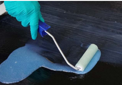
Roller application of SikaBiresin CR169 thix
