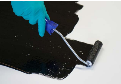
Roller application of SikaBiresin GC155
