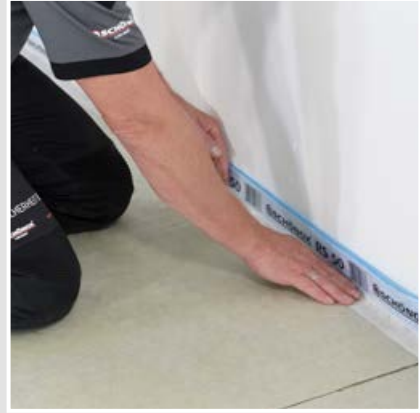
1 SCHÖNOX RS 50 to be installed to all vertical elements.
