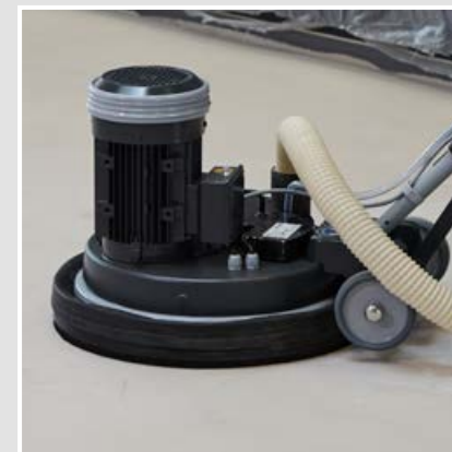
12 The SCHÖNOX HS 50 leveling compound will be fully cured and ready for sanding after approx. 12 hours.
