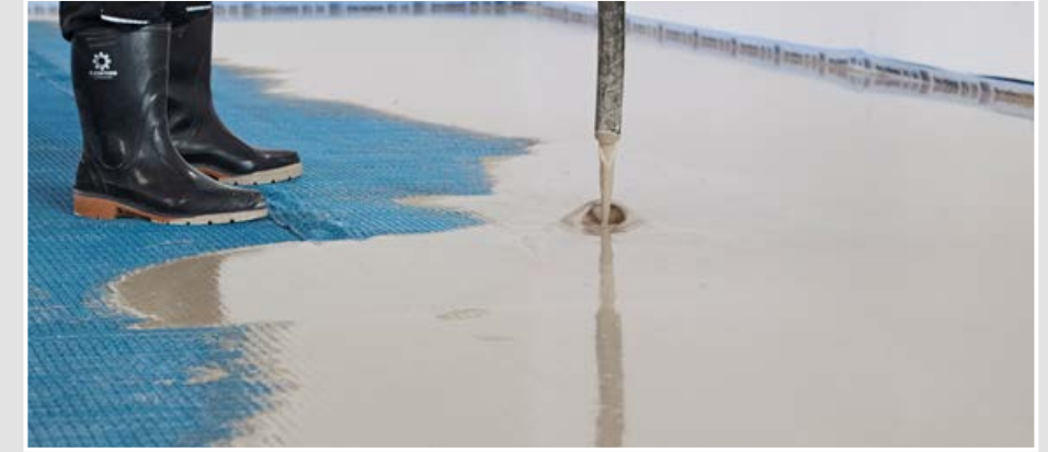
9 Apply SCHÖNOX HS 50 leveling compound. For larger areas, the use of a high power mixer and pump device is recommended.
