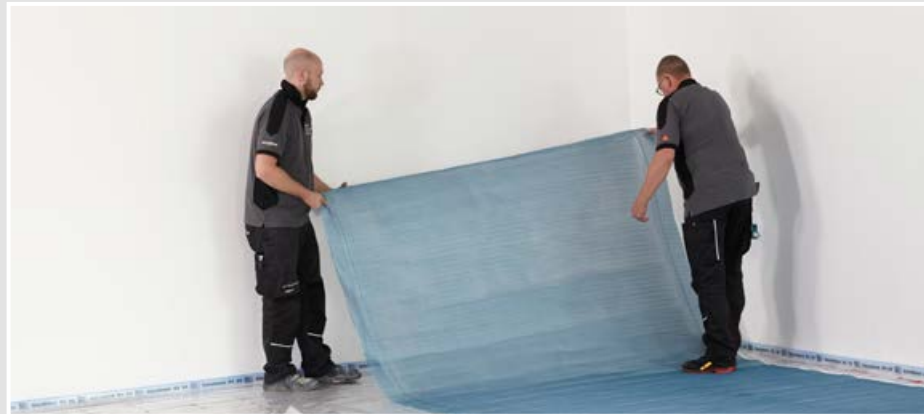
4 Determine the coverage of the SCHÖNOX 3D net according to the size of the room and the required overlap, cut the mesh to size in advance if necessary.
