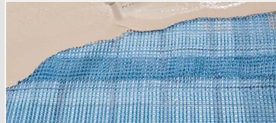
10 IMPORTANT: Do not pour the leveling compound directly onto the overlap area.
