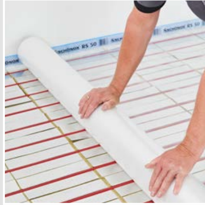
2 Depending on the build-up, a protective PE-foil may be required at approximately 100µ in thickness.
