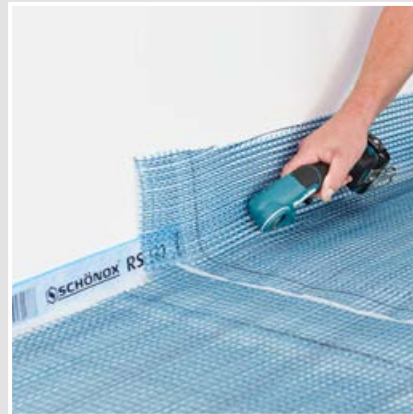
5 Leave a distance of at least 10 mm to the edge-strip.
