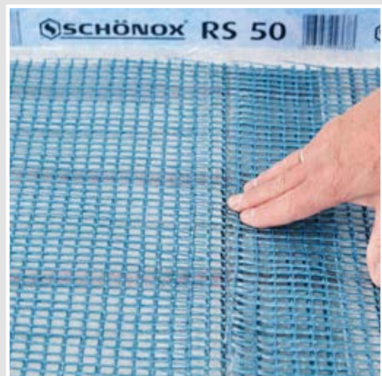
6 The SCHÖNOX 3D net is installed overlapping on the long side.
