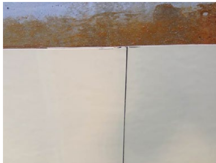
Lap joint with double stripe installation guide: Before bonding, align the top membrane so that the edge sits between the two stripes
