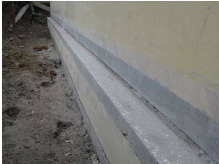
Exposed concrete edges on both sides of the joint
