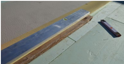
Thermal reforming of the membranes for installing the edge upstand
