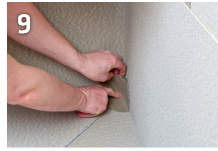
Positioning in the corner without creases
