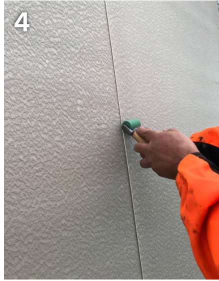
Rolling / rubbing the seam firmly
