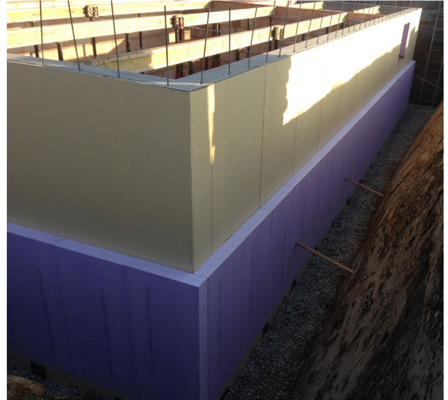
Perimeter insulation with pressure-resistant XPS boards
