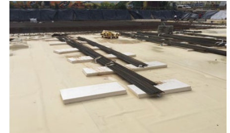
Protective measures for the steel reinforcement
