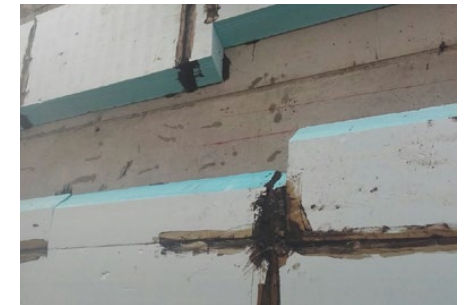
Forming interlocking joints and recesses at a 45° angle in single-sided formwork sections
