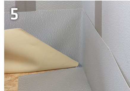
Not cutting right into the corner! Leaving material for inverted pleats
