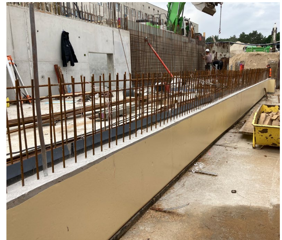
Exposed front face of base plate in a double-sided formwork area
