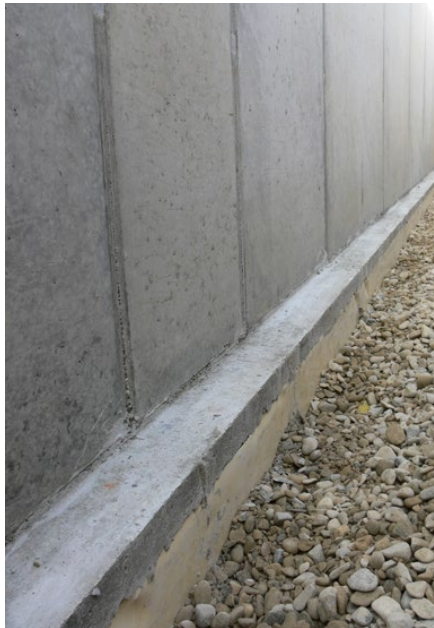
Initial condition: Before applying SikaProof® P-12, formwork joints and the floor slab overhang must be ground smooth, edges chamfered and rounded, plus coves formed as necessary
