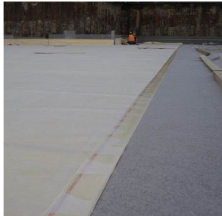
Sheet membranes and geotextiles can be used as a protective layer
