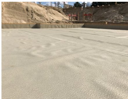
Rippling & distortion due to temperature fluctuations are inherent to the material and do not constitute a defect.
