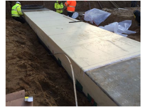
Installation of SikaProof® P-12 on horizontal areas over soffits below
