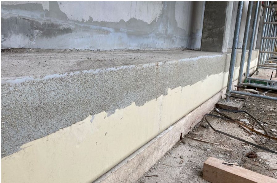
Sanded Sikadur-Combiflex® CF adhesive creates an ideal substrate for bonding liquid applied membranes and coatings
