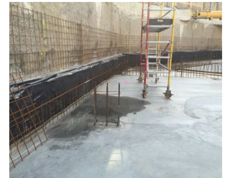
Protected connection area after the floor slab is concreted
