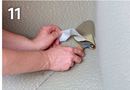
Carefully removing the protective peel liner
