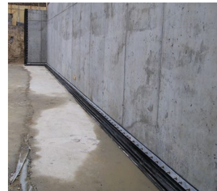
Flanged system using Sika® Tricomer DA 320 KI profile
