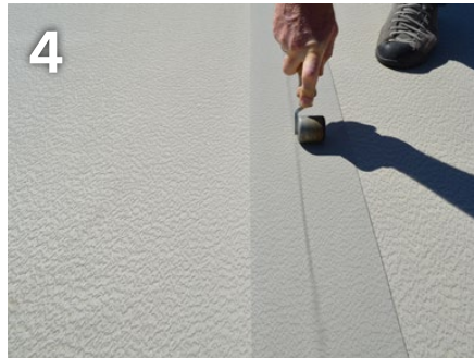
Rolling out the SikaProof® Tape A+N without creases
