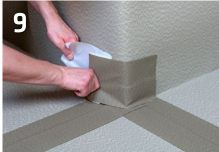
9 Cut and apply an additional section of internal tape to cover the corner detailing
