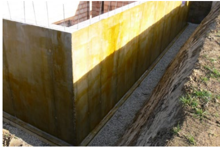
Fully primed surface: Only prime an area that can be installed on the same day
