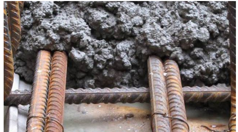
Concreting of SikaProof® A+
