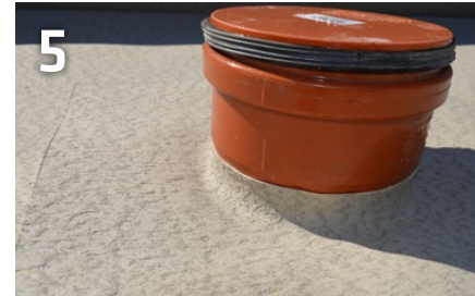
5 Thanks to the thermal flexibility of the SikaProof® A+ collar, it can easily be formed & adjusted to fit exactly.
