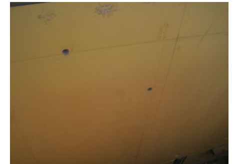
Cutting circular holes 2-3 cm diameter for the tension bars, rather than pushing them through the membrane, to prevent rippling.
