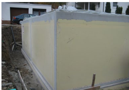
Erecting the wall sections and pouring the core concrete
