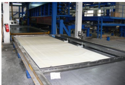
Placing the prepared membrane on the formwork
