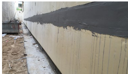
Sikadur-Combiflex® TF taped sealing of the floor-to-wall joint without a floor slab overhang
