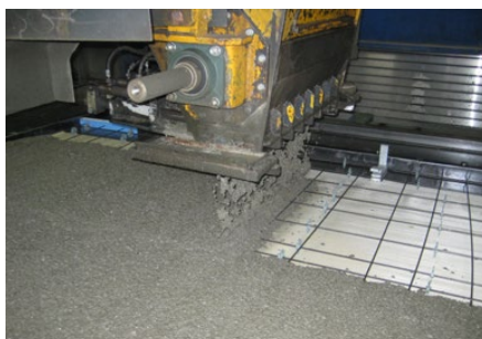
Concreting the precast sections
