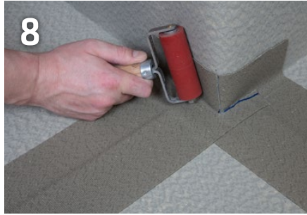
8 Remove the peel liner from the tapes and carefully bond to seal them on the corner with a roller
