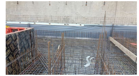
SikaProof® A+ laid through in the slab-to-wall area: The installation substrate in the single-sided wall section is prepared with sufficient height and SikaProof® is extended over the connection reinforcement. A sheet matching the height protects the connection area from concrete contamination
