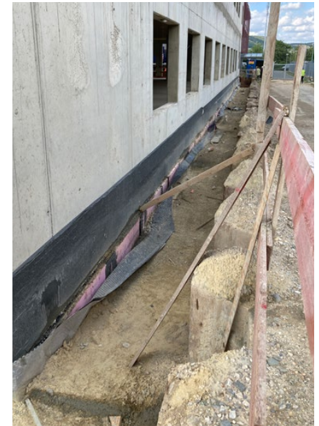
Further waterproofing in the kicker / plinth area with SikaTop®-126 Pro
