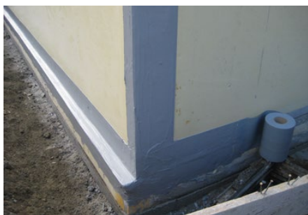
Sealing the joints with Sikadur-Combiflex® TF
