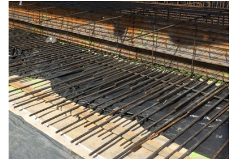
Protect adjacent surfaces with protective sheeting.
