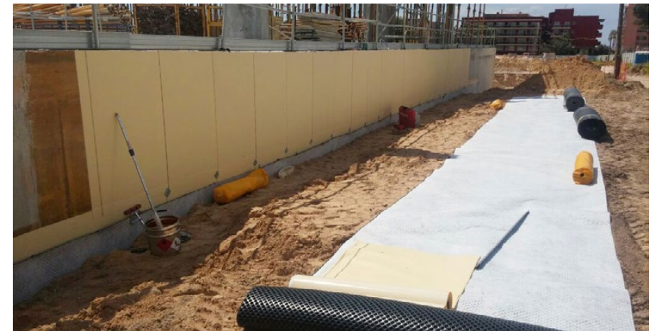
Bridging the construction joint with SikaProof® P-12 and connecting directly to the existing SikaProof® A+ surface, in combination with an additional integral Waterbar
