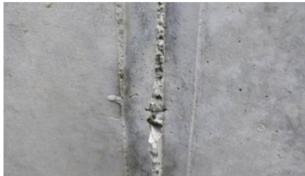
Initial condition: Before applying SikaProof® P-12, formwork joints and the floor slab overhang must be ground smooth, edges chamfered and rounded, plus coves formed as necessary
