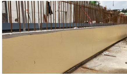
Recessing SikaProof® A+ in the joint area for the subsequent external sealing with the Sikadur-Combiflex® TF System
