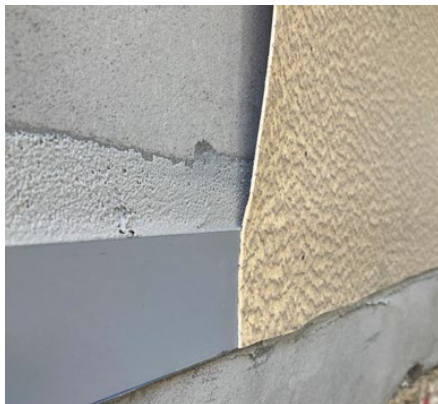
Fixing SikaProof® A+ to pre-bonded Sikaplan® WT Tape-200 welding points or strips. This produces a high-quality, non-penetrating fixing on mineral substrates.
