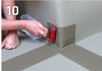
10 Remove the peel liner and carefully roll to bond the additional cover tape in position
