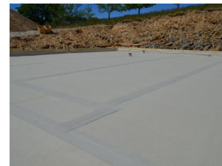
Membrane installed with longitudinal and transverse seams, as well as T-joints
