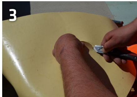
3 Cut out the marked circle with a radius approx. 2-4 cm smaller (depending on pipe's dimension) and heat the membrane on the back around the cutout with hot air
