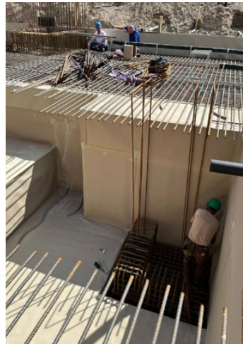
Reinforcement works underway on SikaProof® surfaces with appropriate protective measures
