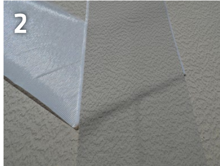
Peeling off the protective liner
