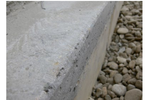
Plinth edge rounded by grinding
