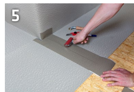
Rolling on the internal tape
