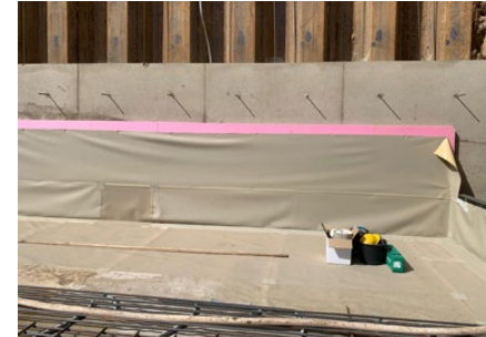
Hanging from clamping rails or nailing strips
