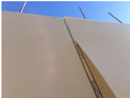
Lap joint with double stripe installation guide: Before bonding, align the top membrane so that the edge sits between the two stripes
