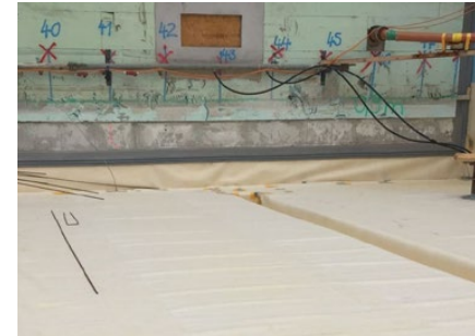
Connection joint to an existing building with Sikadur-Combiflex® TF Profile DFT 330/3 KFV
