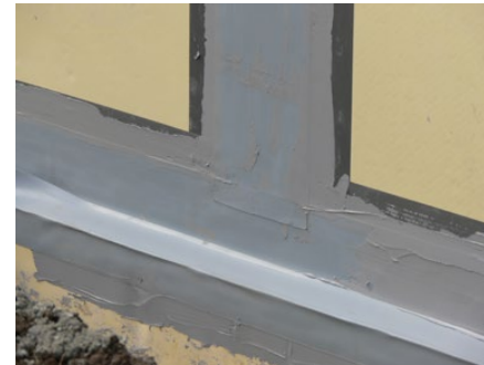
Application of the Sikadur-Combiflex® TF system and connections to the SikaProof® membrane surface.
