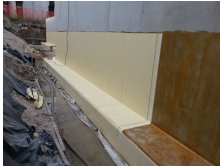
Quality concrete is crucial for the performance and efficiency of this method
