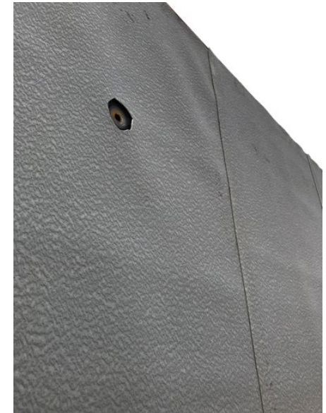
Always locate horizontal joints in areas with double-sided formwork following the umbrella principle
