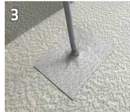
3 Cutting the SikaProof® Tape A+ to size, drawing it over the electrode and fixing it onto the waterproofing membrane.
