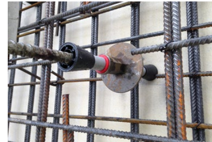
Installation of the tension sleeve in the formwork
