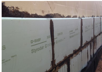
Full-surface bonding of Perimeter Insulation
