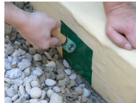
Secure T-joints with SikaProof® ExTape-150, pressed on firmly with a hand roller
