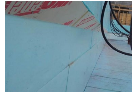
Forming interlocking joints and recesses at a 45° angle in single-sided formwork sections
