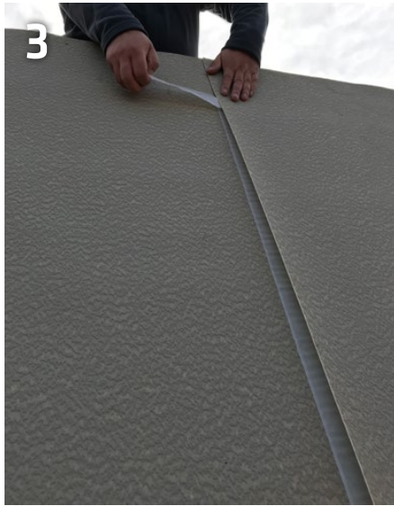
Peeling off the protective strip
