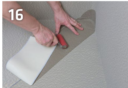
Rolling and firmly rubbing the interior tape for a full bond to the membrane with a pressure roller
