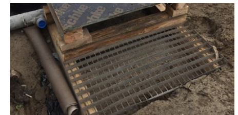
Strictly defined access by installing a grids to form a clean walking zone
