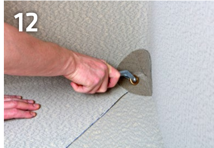
Carefully rolling and rubbing it firmly to bond the piece in position on the membrane in the corner
