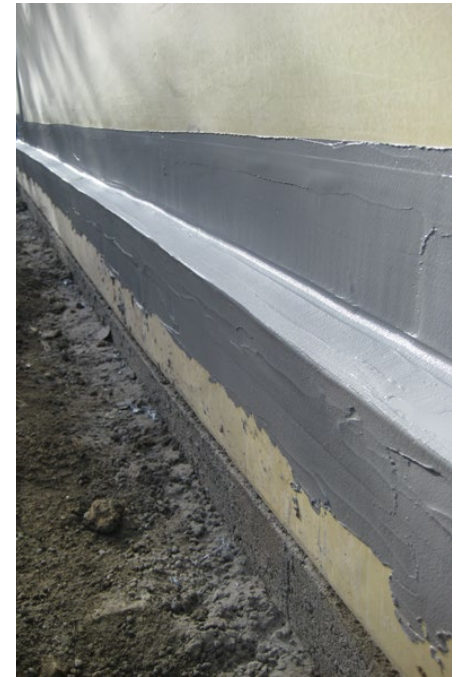
Finished Sikadur-Combiflex® TF system installation and connection to SikaProof® membrane
