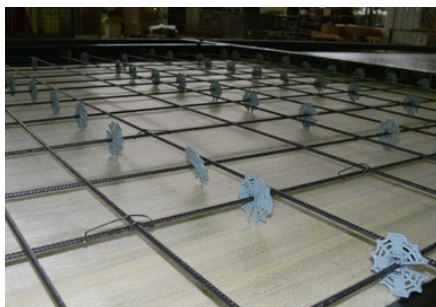
Installation of the reinforcement
