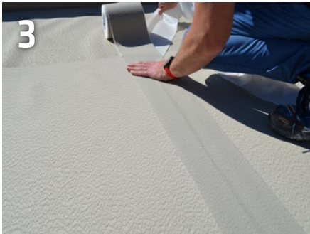
Applying the tape
