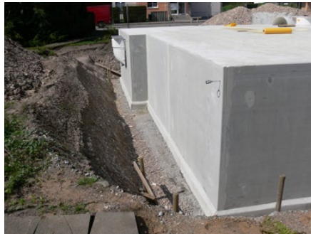
Watertight basement with precast concrete walls
