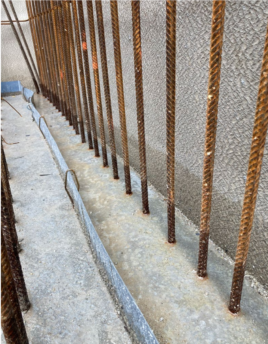
Result: a clean construction joint achieved by using a protective sheet
