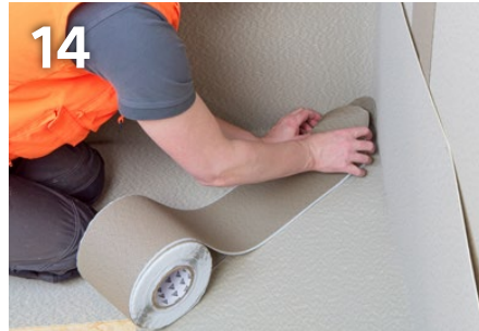
Positioning the interior tape
