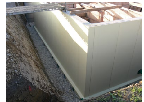
Visual inspection and quality assurance before applying protection and backfilling the area
