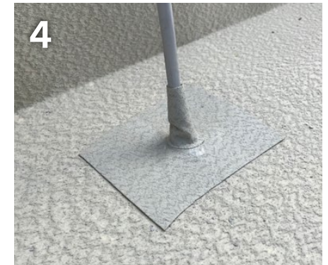
4 Cut a second piece of SikaProof® Tape A+ to size and use it to seal the transition
