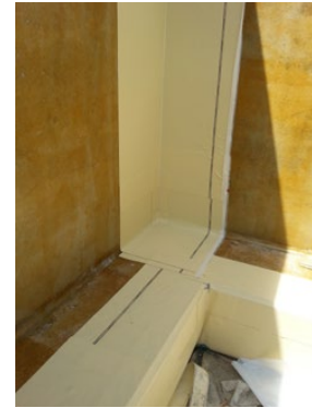
Forming internal corners / corner combinations
