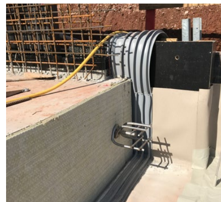
Expansion joint forming with Sikadur-Combiflex® TF joint tape profile DFT 330
