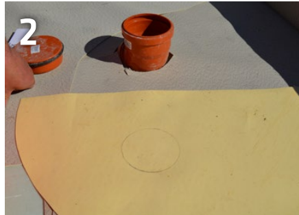
2 Prepare the patch and mark the circumference of the pipe penetration in the centre
