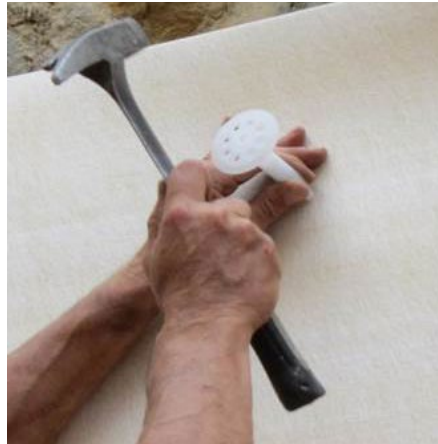
Fixing SikaProof® membrane with anchors into perimeter insulation
