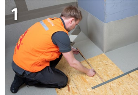
Cutting and laying the membrane
