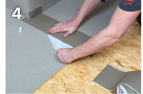
Cutting the internal tape to size, removing the liner, and bonding it in position firmly with a roller
