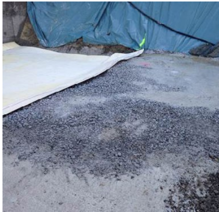
Inadequate substrate quality
