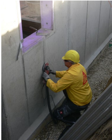
Grinding formwork joints
