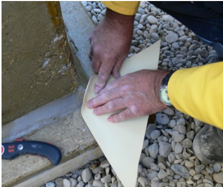
Inserting fitted pieces
