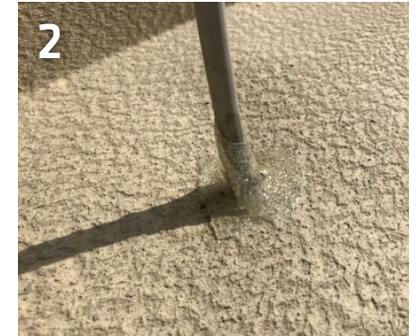
2 Seal the transition from bonding layer to electrode with SikaProof® Sandwich-Tape as shown
