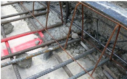
Contamination from grout loss and leaks around formwork must be prevented, with any seepage removed and cleaned off immediately whilst fresh
