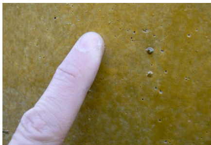
Finger test: Before installing SikaProof® P-12, the primer must be dry to the touch
