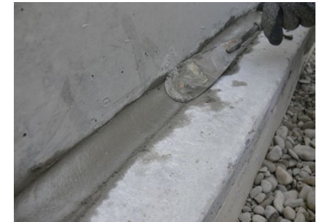
Forming a PCC mortar cove
