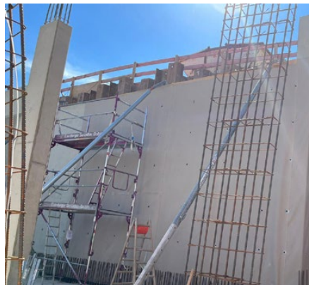
Fixing SikaProof® membrane with anchors into perimeter insulation
