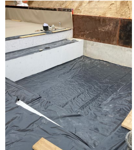
Floor slab installation on slip membrane (PE film)
