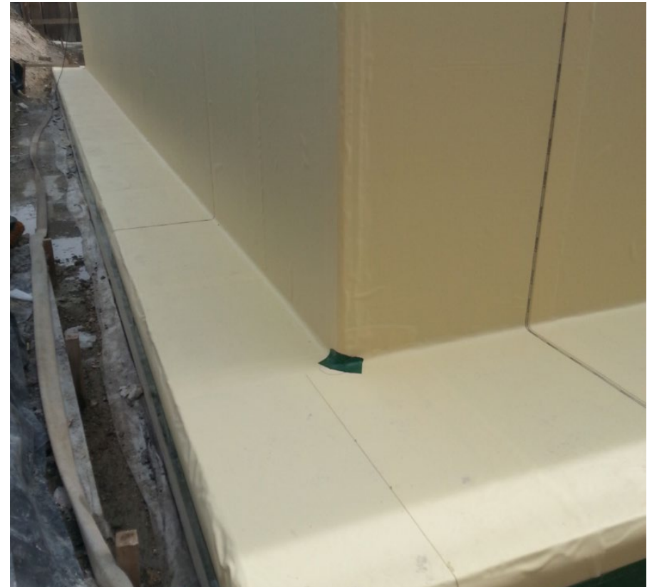
Final sealing and securing of the detailing in accordance with section "4.6 Corner Detailing"
