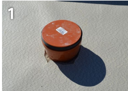
1 Lay the membrane and roughly cut out a hole for the pipe penetration
