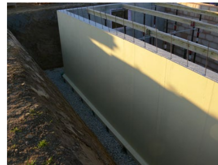
Visual inspection and quality assurance before applying protection and backfilling the area
