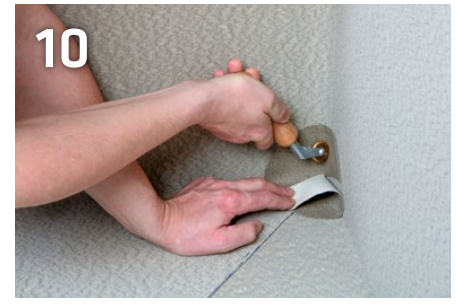
Carefully rolling and forming it with a roller
