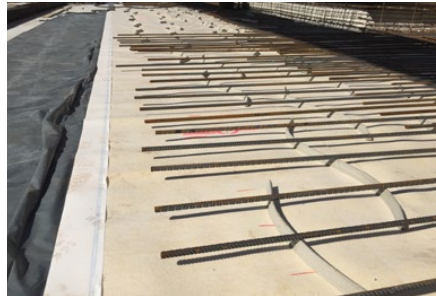
Extend the FBV membranes in the connection area, to beyond the longest connecting reinforcement.
