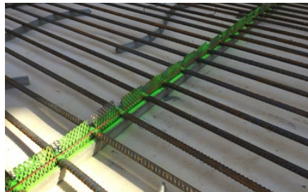
Reinforcement spacers are designed to provide an effective solution to preventing leaks and contamination of joint connection areas
