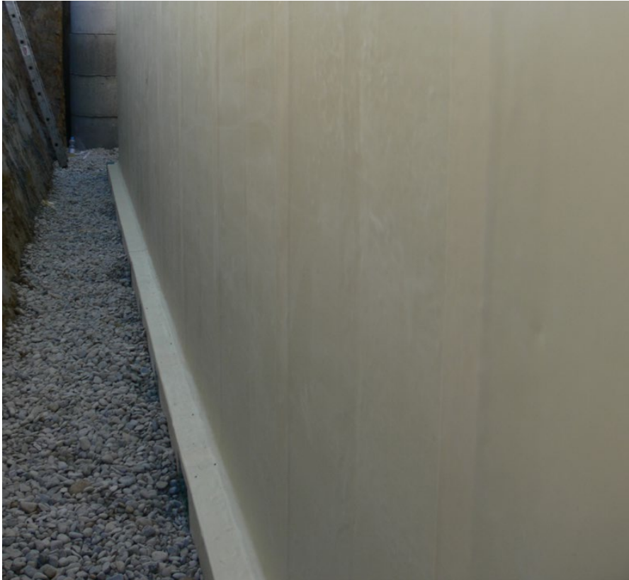
The tensioning points are covered over the entire surface after sealing with the plugs included in the system
