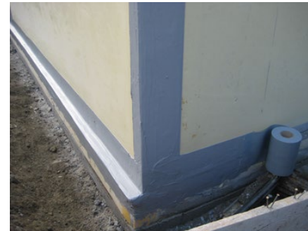
Maximum flexibility when designing shaped pieces for intersections, etc. due to thermal weldability
