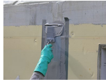
Application of the Sikadur-Combiflex® TF system and connections to the SikaProof® membrane surface.
