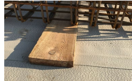
Support timber for the temporary storage of a pre-tied reinforcement cage
