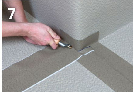
7 Carefully rolling to form the internal tapes in position on the corner
