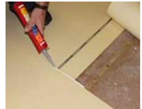
For pressures over 5 m head: additionally secure the offset of T-joints and detailing joints with sealant (e.g., Sikaflex® 11FC), applied in beads (2–3 mm), then pressed and rubbed in firmly with a hand roller
