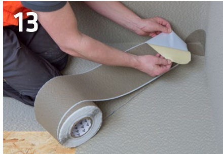
Cutting the interior tape to size
