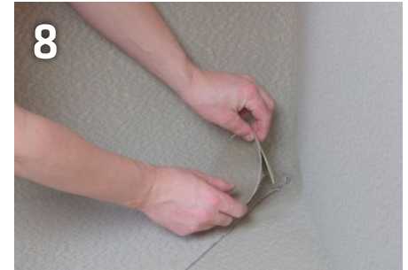
Forming into a cone shape to fit the corner
