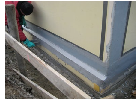
Application of the Sikadur-Combiflex® TF system and connections to the SikaProof® membrane surface.
