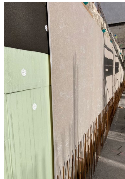
Installation on perimeter insulation in single-sided formwork sections
