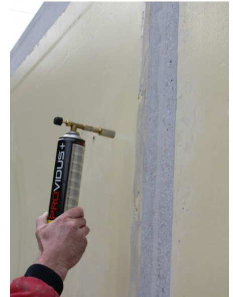
Briefly torching the surface of the SikaProof® membrane in the lap area before applying the Sikadur-Combiflex® TF system
