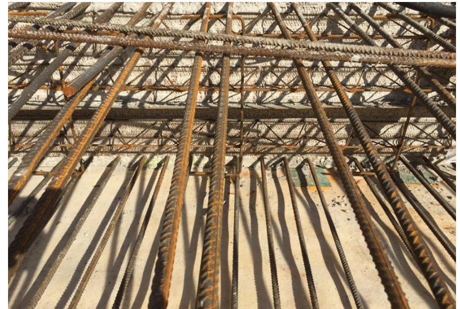
Result: Perfectly formed construction joint: The spacer under the lowest reinforcement layer is clearly visible and the adjacent SikaProof® A+ is free of any unwanted contamination
