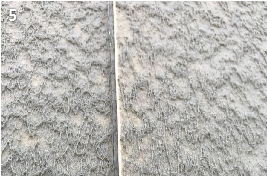
The seam must be fully bonded over the entire bonding areas, with no voids or capillaries
