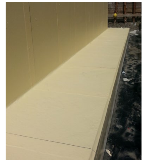
Horizontal areas with wide floor slab overhangs
