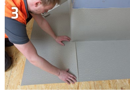
Fitting the sealing piece in position
