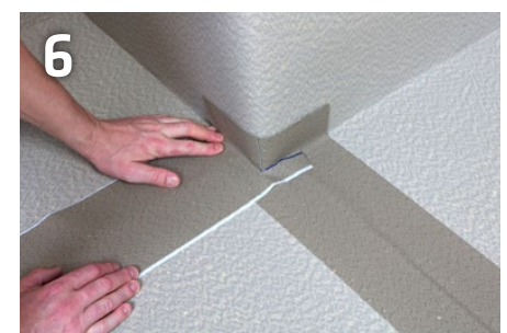
Repeat with the 2nd piece of internal tape
