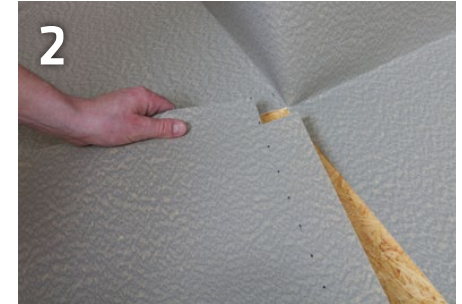
Cutting and making a sealing piece to size
