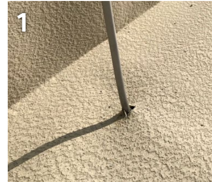
1 Cut out and heat the SikaProof® A+ membrane to fit and draw it over the electrode
