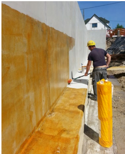
Applying SikaProof® Primer-01
