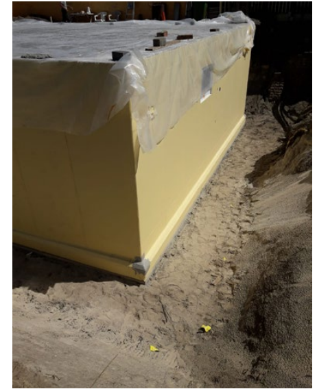
Further waterproofing work with SikaProof® P-12
