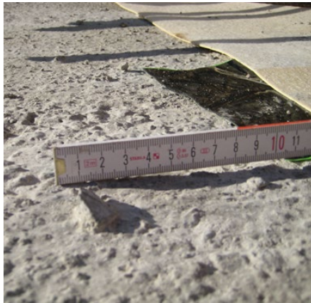
Knock off any protruding sharp edges, brush away and remove loose and friable particles
