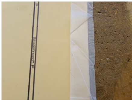
Additional bonded edge at a longitudinal joint: Remove the protective liner before bonding the membrane
