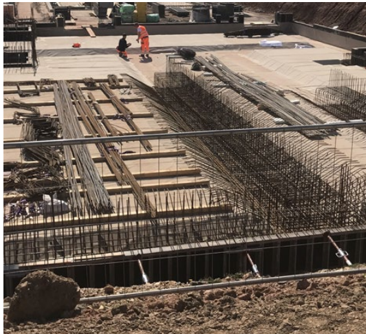
Reinforcement works underway on SikaProof® surfaces with appropriate protective measures
