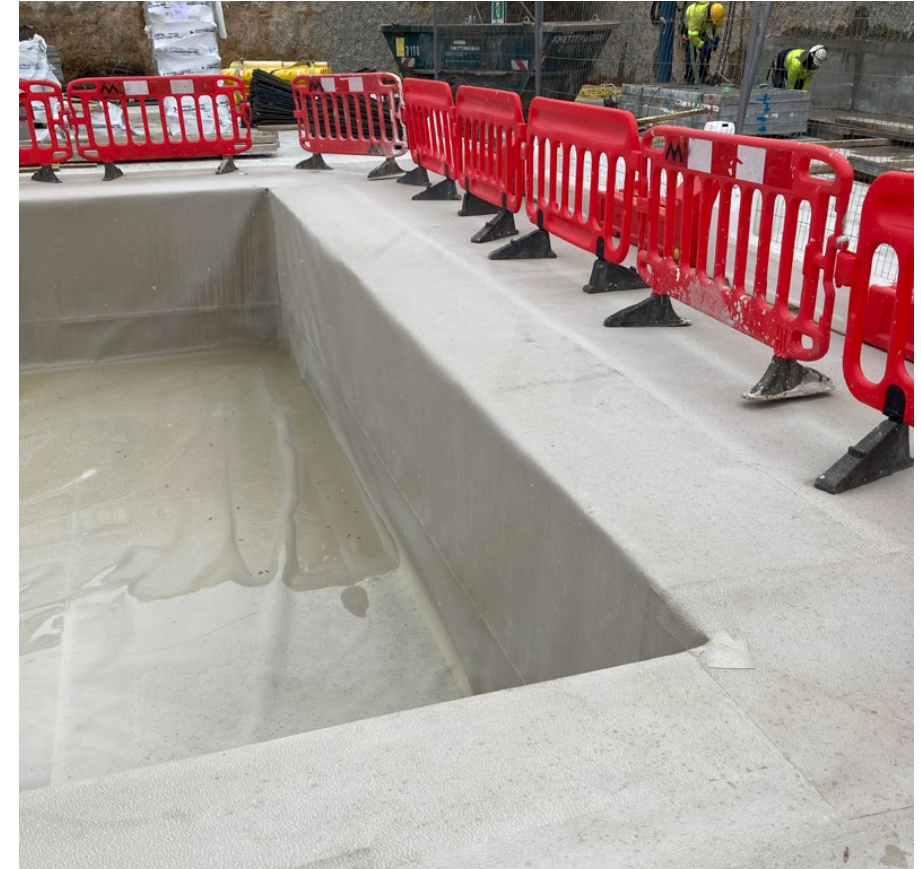
Corner detailing in an elevator pit
