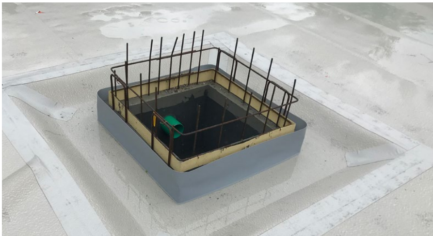
An example of sealing a precast sump pump with the Sikadur-Combiflex® TF System
