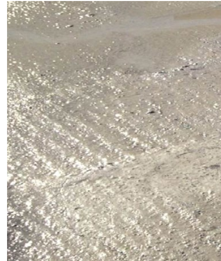
Lean concrete blinding, poured and vibrated to allow the aggregate to settle for a good surface finish
