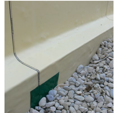
Finished sealed T-joints
