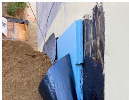
Installation of perimeter insulation with solvent-free, 2-component, PMBC adhesive coating
