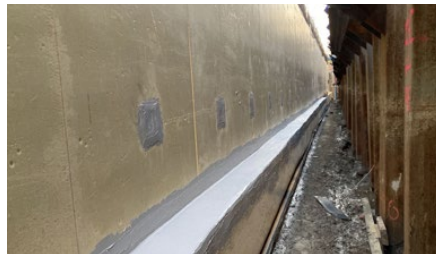
Sikadur-Combiflex® TF taped sealing of the floor-to-wall joint with a floor slab overhang
