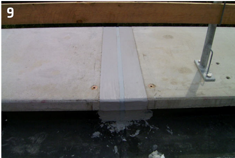
LFT waterbar profile in visible area of a bridge coping
