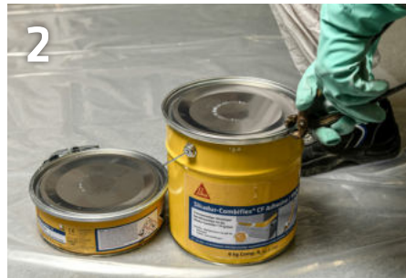
Open the container carefully with pliers (use the breakaway line on the snap ring).
