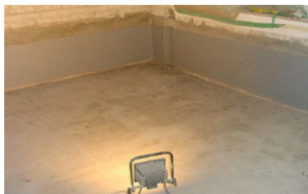
Jointing sealing construction as new inner trough for the renovation of an existing basement
