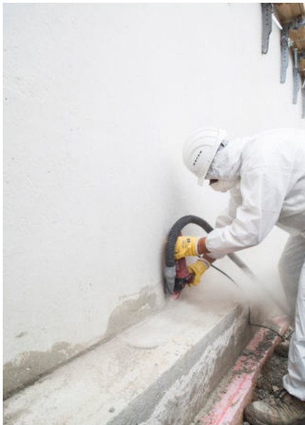
Substrate preparation by grinding the concrete surfaces
