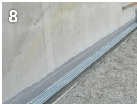
Finished applied DFT waterbar profile
