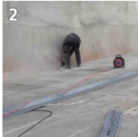
Preparation of substrate by grinding the subsequent bonding surface
