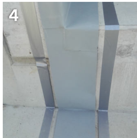
Apply tape to the edge of the sealing in the visible areas
