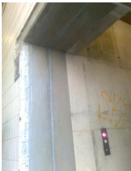
Renovation of an expansion joint - in this case a supporting structure by means of drag plate flashing is required.
