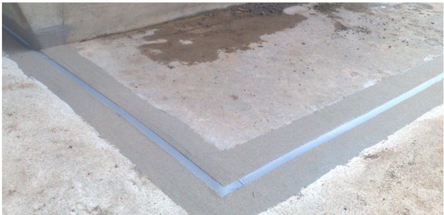
Sealing an expansion joint
