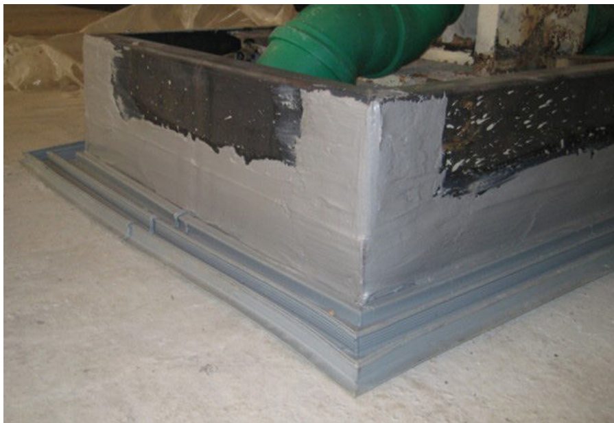
Connection of a new base plate to steel supports by sealing with a DFT waterbar profile
