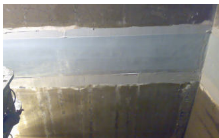
Renovation of a leaking construction joint
