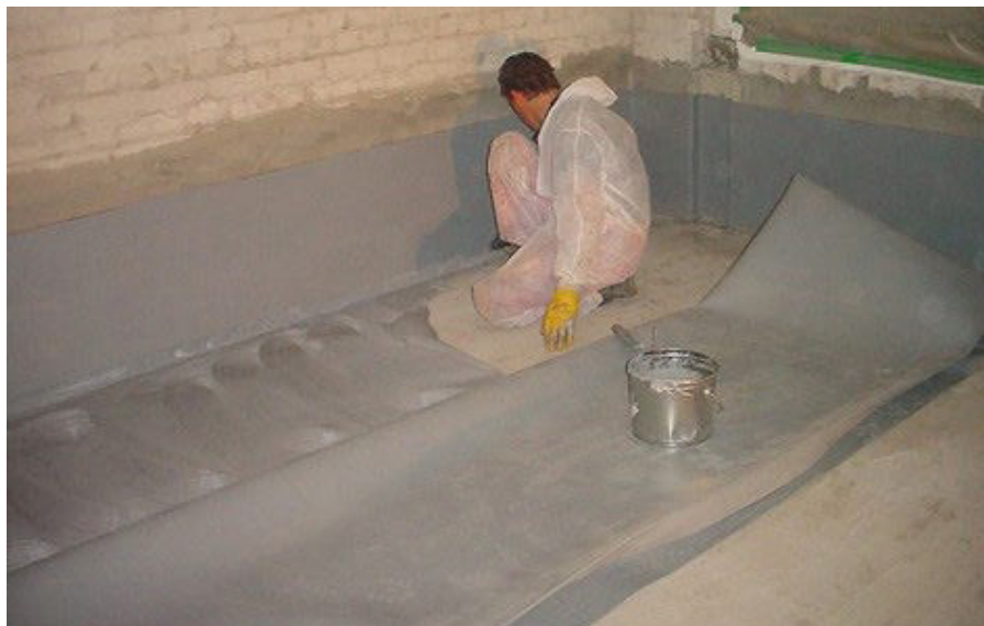
Jointing sealing construction as new inner trough for the renovation of an existing basement
