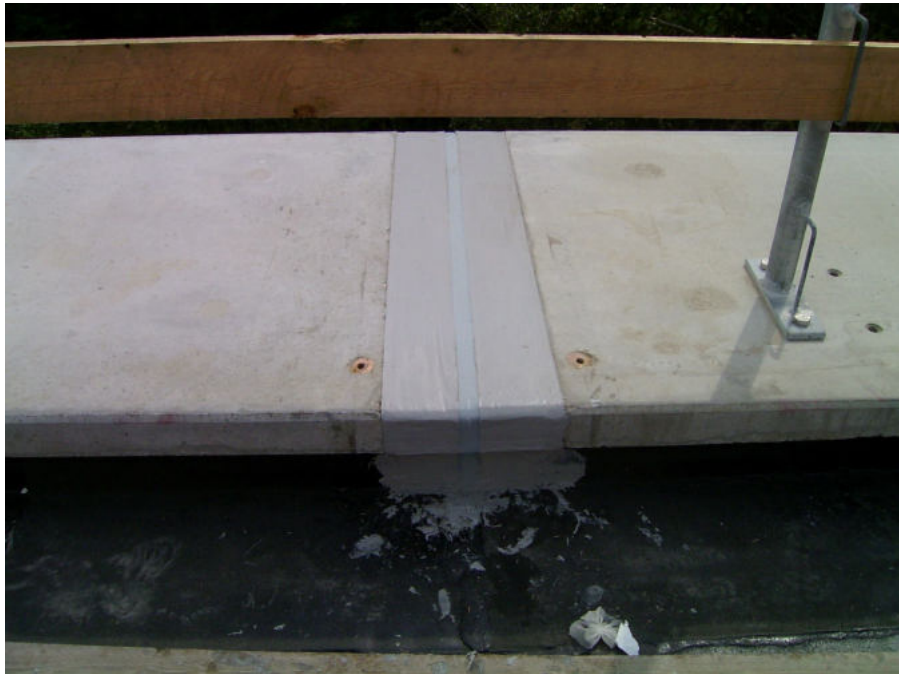
This configuration can be used for waterproofing on bridge constructions and complies with the specifications of the BASt standard drawing FUG 4 sheet 2.
