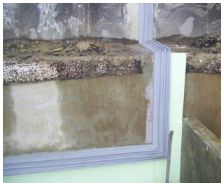
Sealing a connection joint on an existing structure with FAT130/3 KF profile
