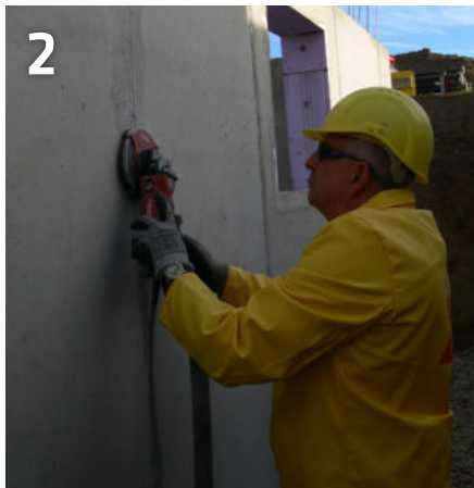
Prepare substrate by grinding with concrete grinding disc
