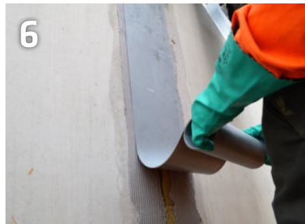
Lay the 2 mm jointing tape into the fresh adhesive layer near an expansion joint
