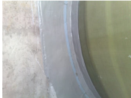
Sealing of a GRP pipe penetration
