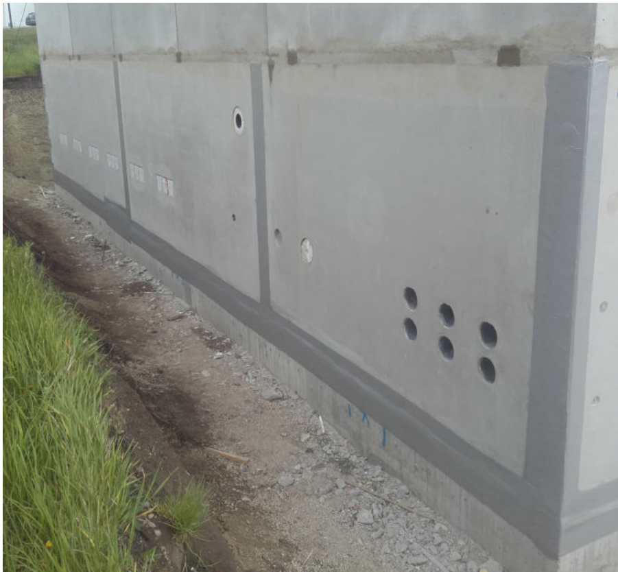
Sealing of construction joints based on the example of a precast basement
